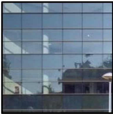
GREY TINTED LOW-E GLASS TO TOWER FACADE
